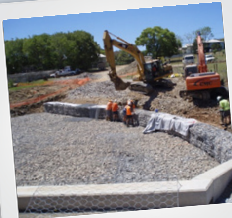
Work crew building gabion walls in Commissioner's Gully
